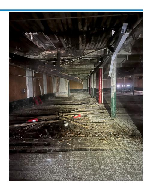
In addition to the exterior openings there is interior damage to floors and the roof that make entering the building with poor visibility unsafe
